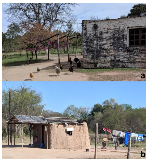
Figure 2. Households with (a) brick walls and (b) adobe walls in the neighborhoods surrounding Pampa del Indio, Chaco, Argentina. July 11, 2018.
